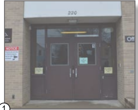
① HOLLOW METAL DOORS & HOLLOW METAL FRAME
